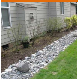
Modified French Drain
