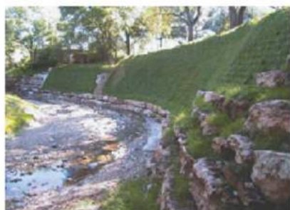
Green Gabion Wall
