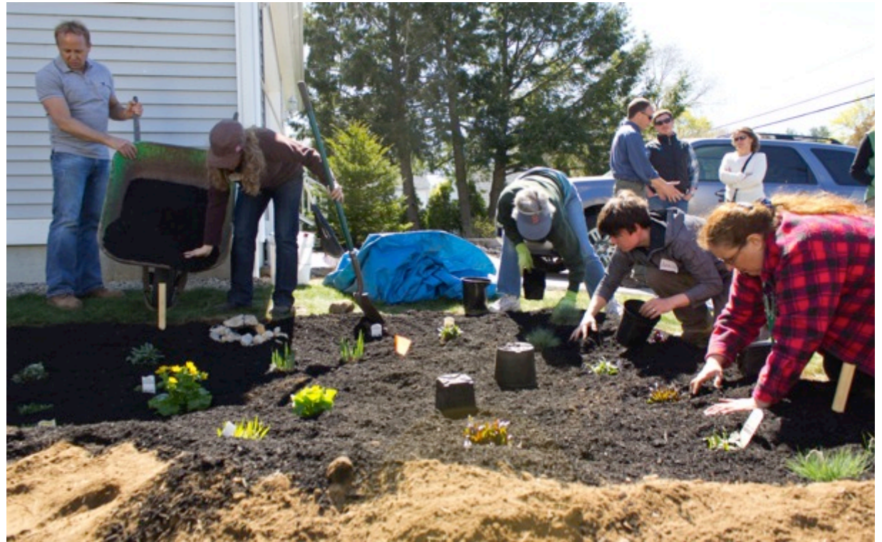
Rain gardens collecting water diverted from downspouts
