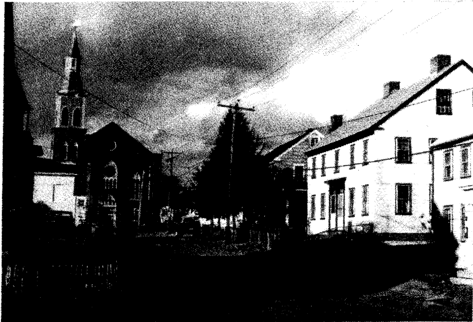
existing conditions, mechanic street
