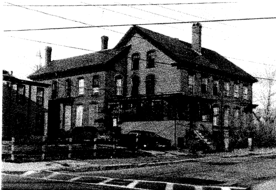
housing - school street
