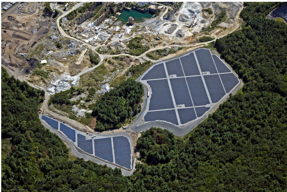
Westford Solar Park
