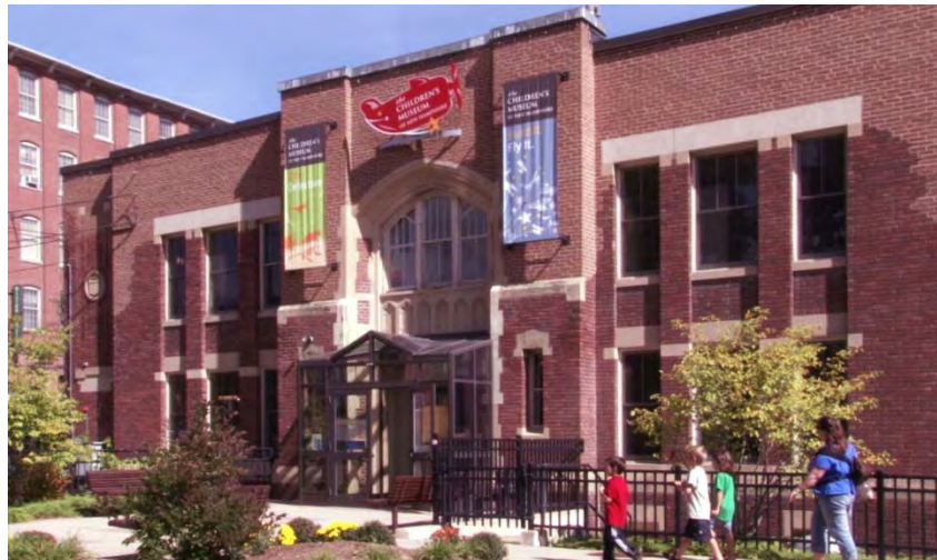
Figure 13: In 2007 the City of Dover worked with the Children's Museum of New Hampshire to move into Dover's downtown. The museum rehabilitated the City's former recreation center into a 60,000 square foot plus museum with expanded cultural amenities.
