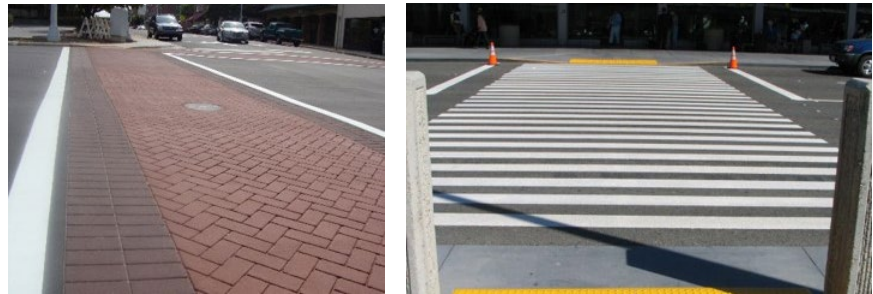
Figure 19: Example crosswalk paving patterns and materials
