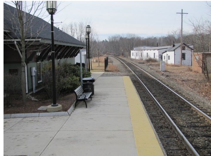
Low level platform — looking west
