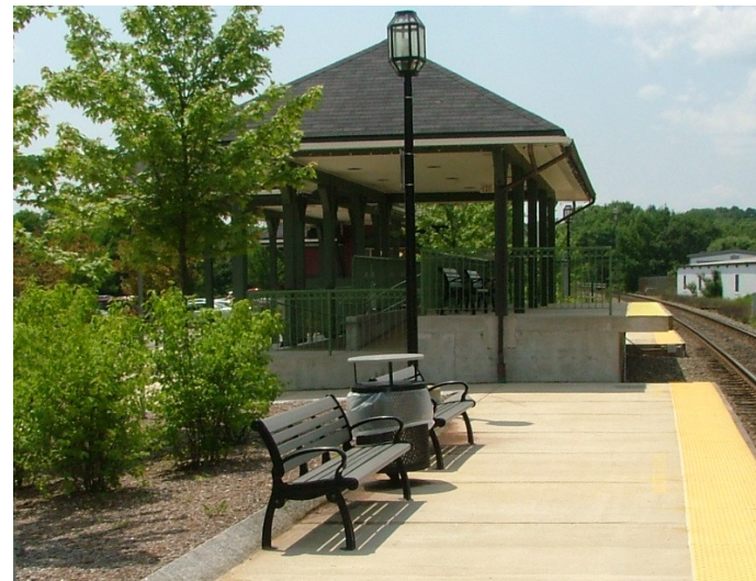
High level platform — looking west
