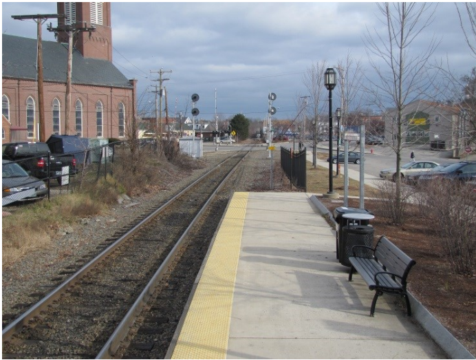
Low level platform — looking east
