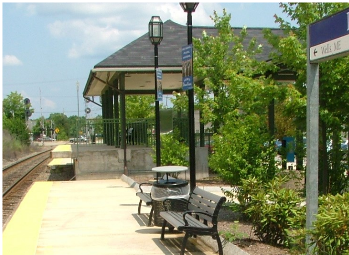
High level platform — looking east
