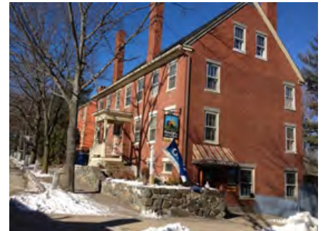
Figure 44. Specialty Businesses Located in Attractive Historic Structures
