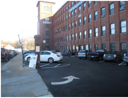
A smaller parking lot in downtown that lacks any frontage planting or walls/fences along the street to buffer and soften the appearance.
