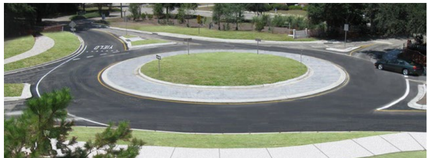
Figure 20: Typical mini-roundabout configuration
