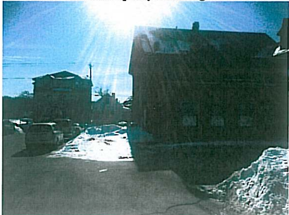
Northwest Entrance looking South
