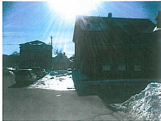
Northwest Entrance looking South
