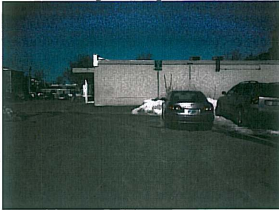
West End of Property Looking North- Janeto's Shopping Plaza
