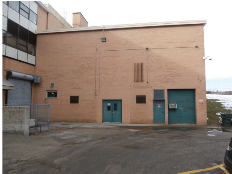
5. North side of 1967 building – low roof locker room wing.
