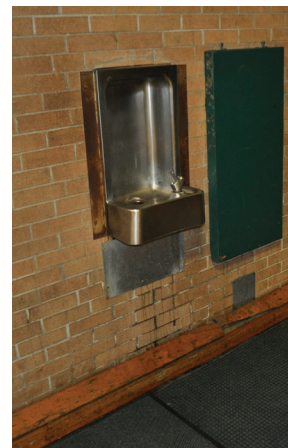
Drinking Fountain, Aged Base Board & Cracking CMU
