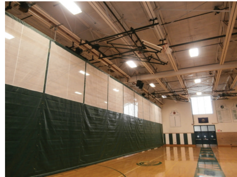
7. Gymnasium, long span open web joists, tectum roof deck on bulb tees.
