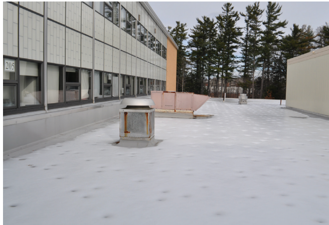
View of Roof with snow cover
