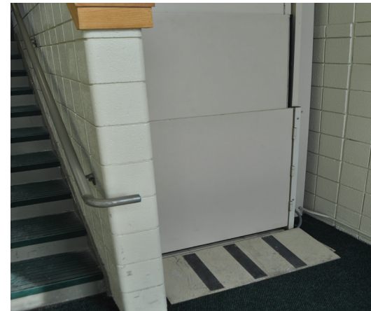
Lift at CTC Entrance
