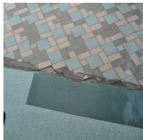
Missing Expansion Joint at 2002 Addition
