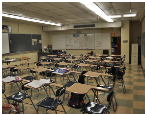
Typical Classroom - Asbestos Tile Floor
