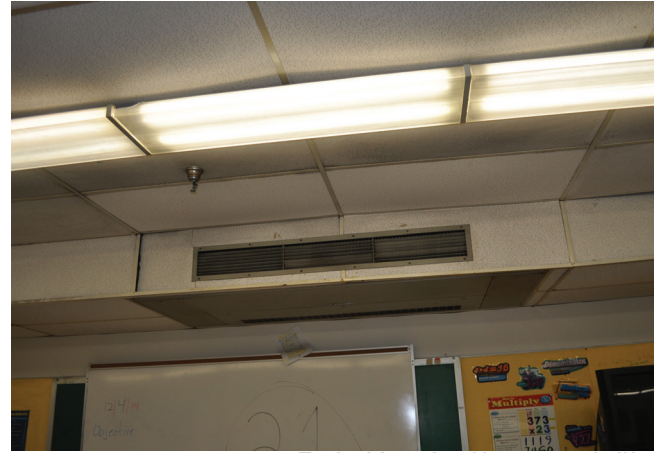
Typical Interior Classroom Ceiling
