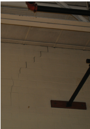
Drinking Fountain, Aged Base Board & Cracking CMU
