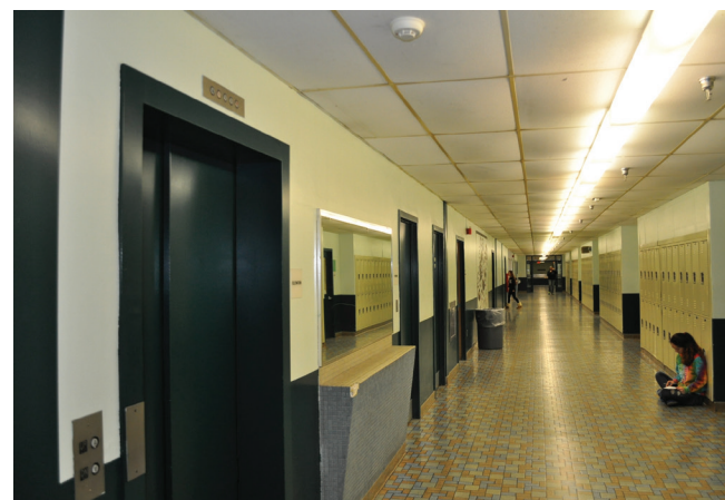
Remotely Located Elevator
