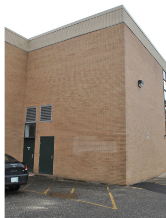
Visible Efflorescence
