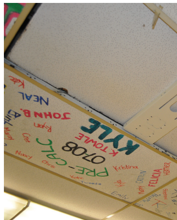
Typical, Painted Ceiling Tiles
