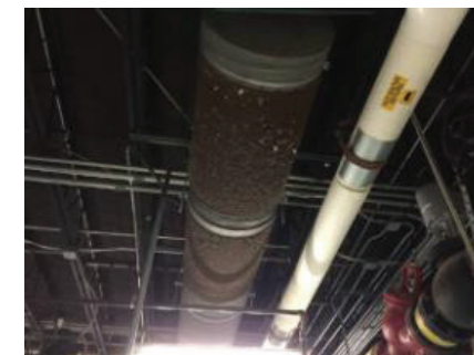
Combustion Air Perforated Supply Diffuser
