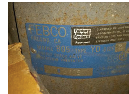
Double check valve assembly
