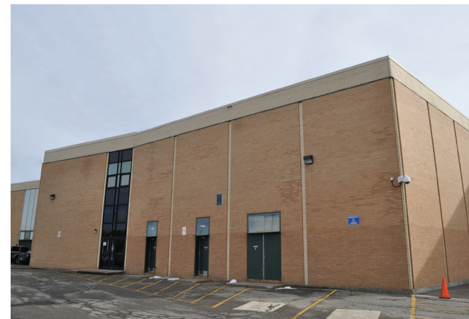
Exterior Wall System 1 - Brick Veneer
