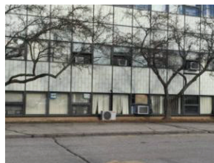
Window AC Units
