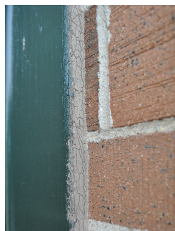
Cracked Sealant
