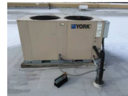
Administration Area ACC Unit
