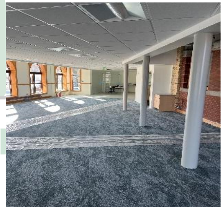
Figure 18: Only finishing touches left on this floor.
