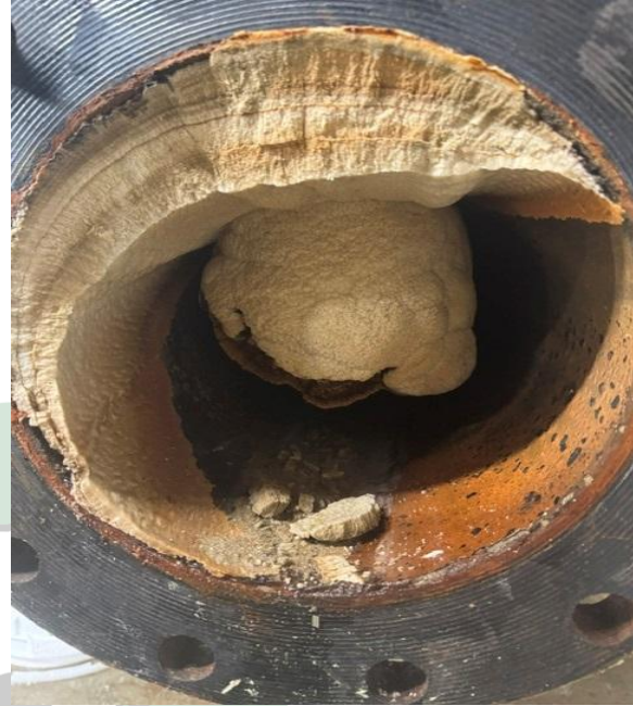
Figure 14: The start to material removal.
