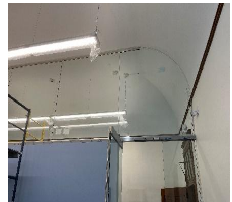
Figure 19: The start to permanent power being installed.
