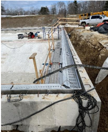
Figure 21: New gutter installation at the Jenny Thompson Pool.
