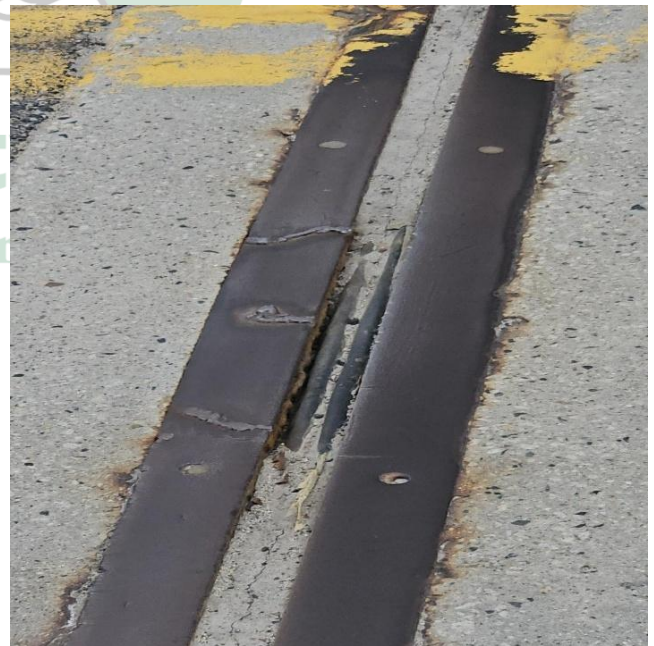
Figure 9: Welding repair on the bridge expansion joint on Chestnut Street.
