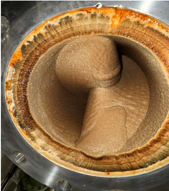
Figure 13: Calcium buildup, almost as strong as concrete.
