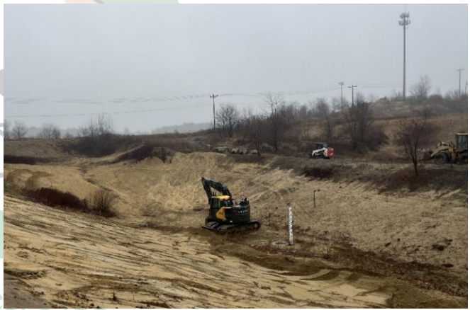
Figure 11: Cleaning the recharge basin.
