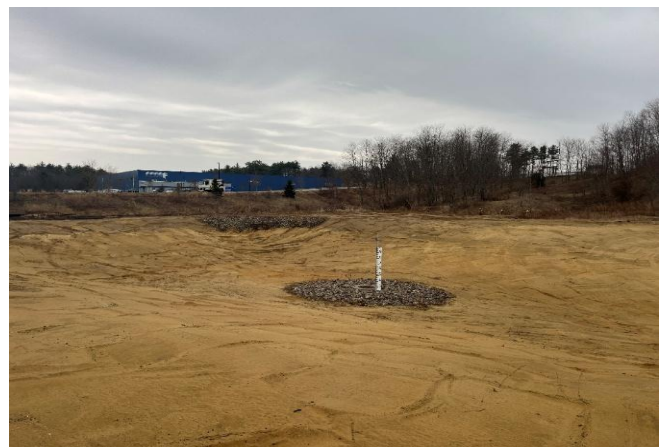
Figure 12: Basin work completed and is working at its best again.
