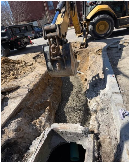
Figure 2: Drain line replacement in the orchard Street parking lot.
