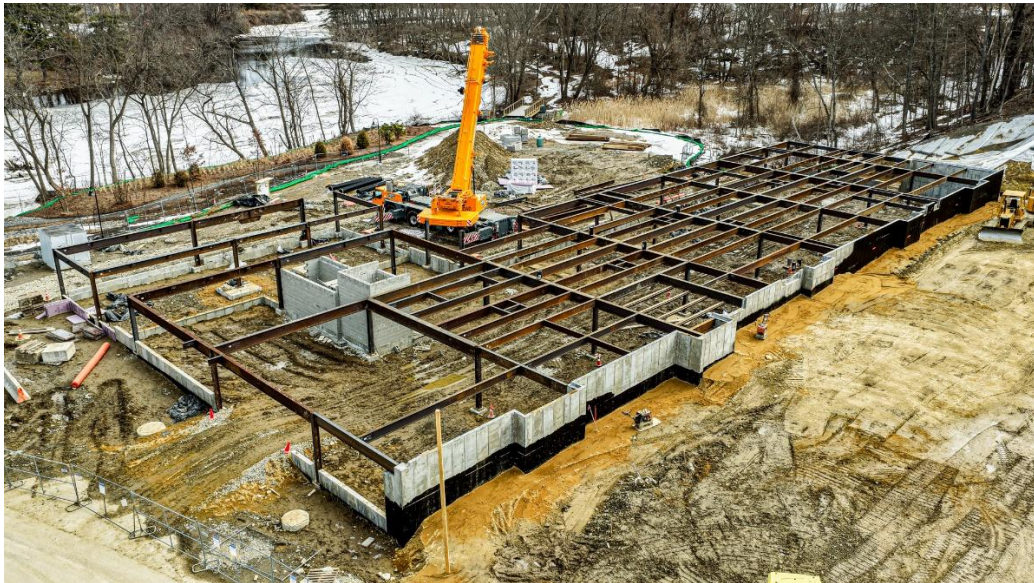
Figure 5: First floor structural steel is set for Building F.
