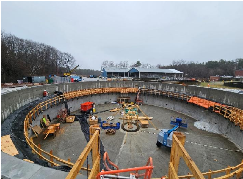
Figure 24: Secondary Clarifier making great headway.
