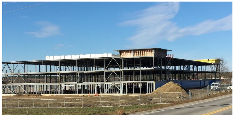
Figure 6: Bluebird Storage Facility on Littleworth Rd.
