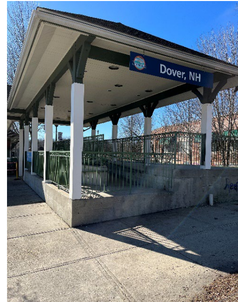
Figure 11: Dover Transportation Center Column Replacement.
