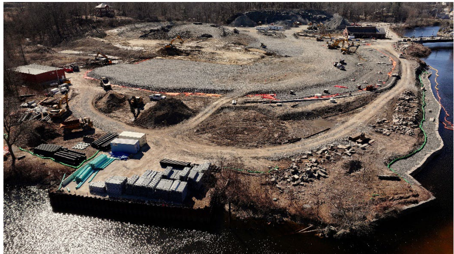
Figure 8: Parcel 1-4 and 1-5 subgrade work at the Waterfront.
