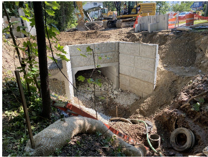
Figure 1: Installation of new precast concrete box culvert below Hough Street.
