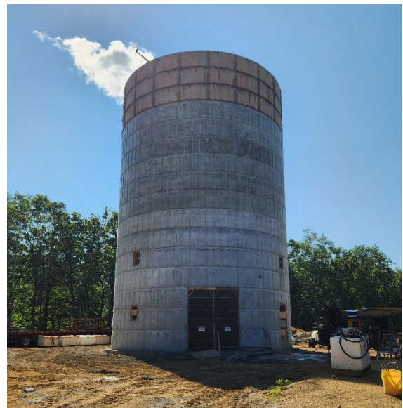
Figure 5: New elevated tank pedestal continues to rise.
