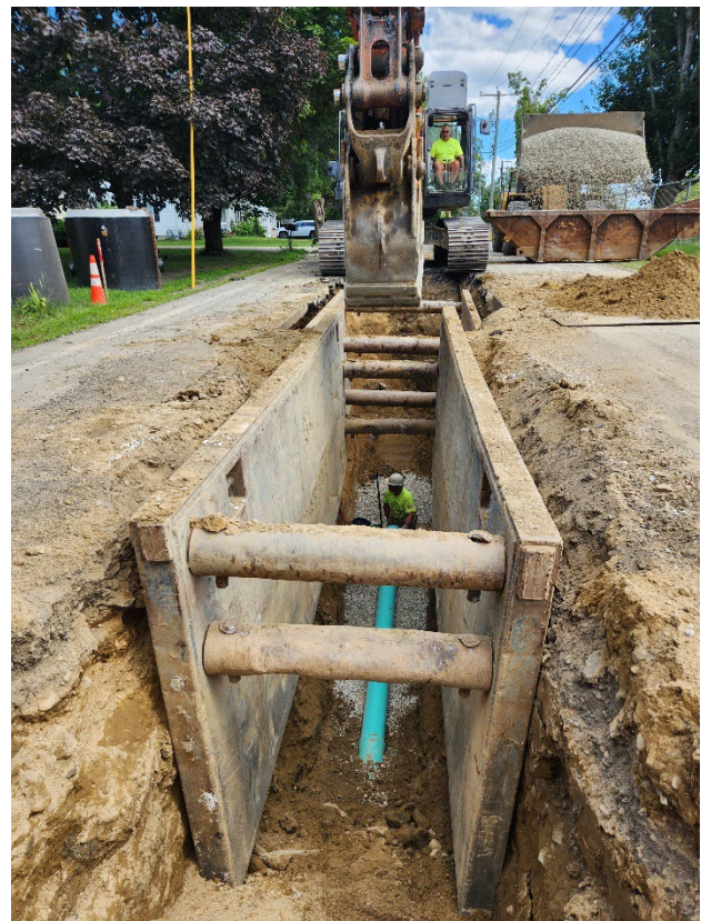
Figure 4: Court Street Emergency Sewer Repair.
