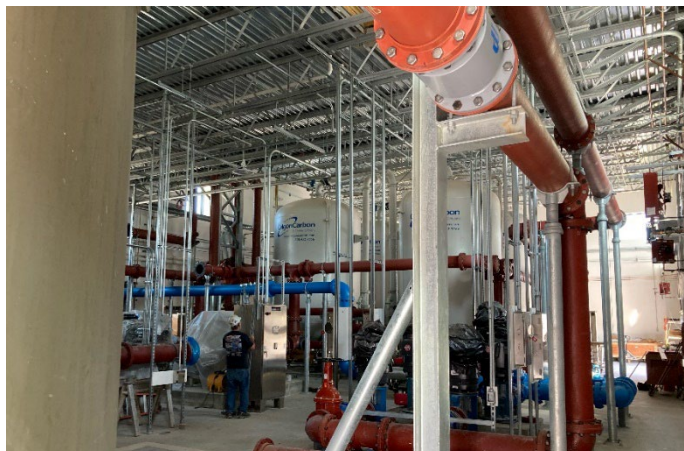
Figure 2: Interior fit up at the new Pudding Hill Water Treatment Plant.
