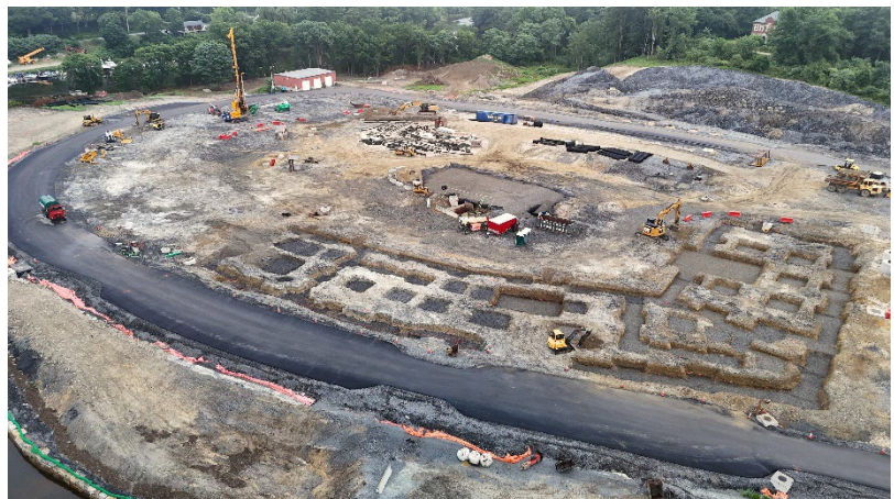
Figure 5: Waterfront foundation progress on building C.
