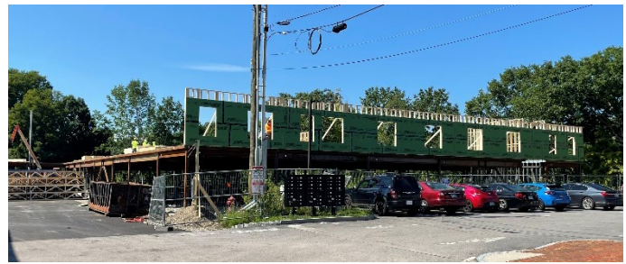
Figure 9: 2 Grove Street is beginning to rise.
