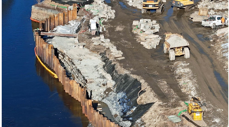
Figure 5: Granite Wall Construction along the waterfront.
