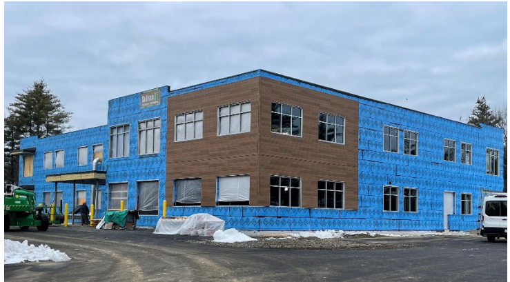
Figure 9: 7 West Durham Road Medical Office.
