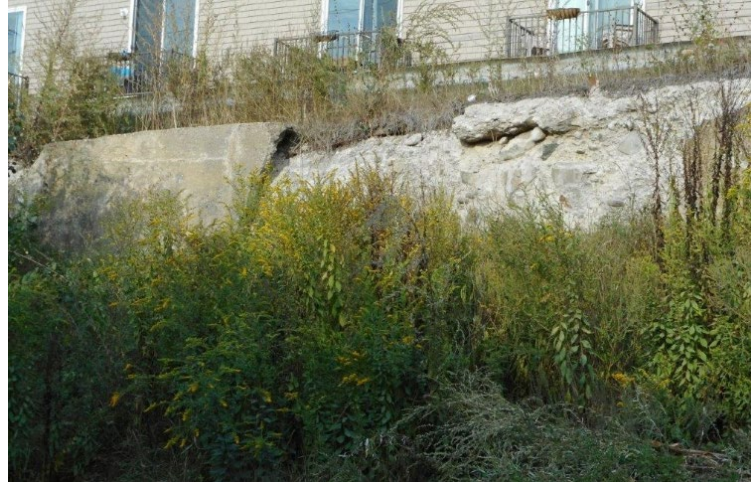
Figure 3: Existing Portland Ave Retaining Wall
