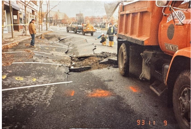
Figure 6: Water main break in Central Ave near Second Street from November 9, 1993.
