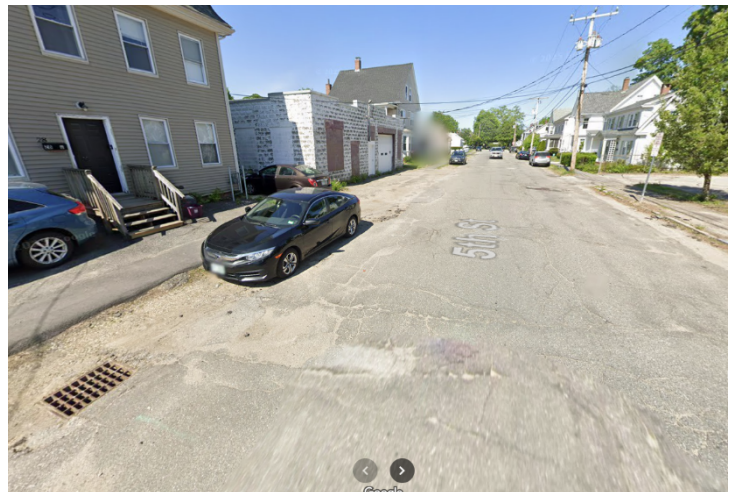
Figure 5: Fifth Street Deterioration in May 2023 prior to reconstruction (via Google).
