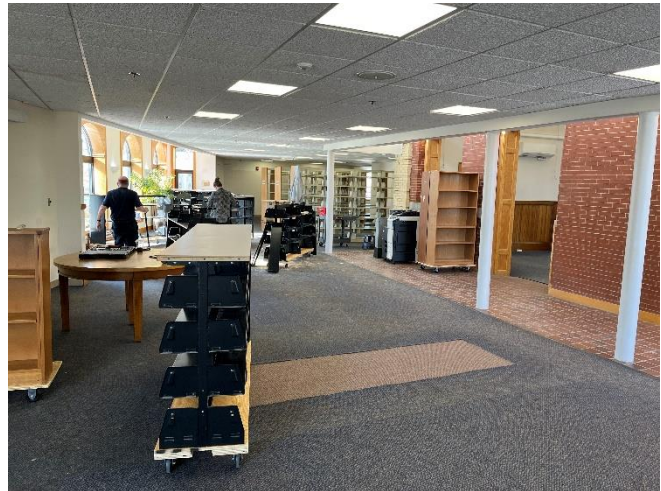
Figure 14: The library renovation is about to start ramping up.
