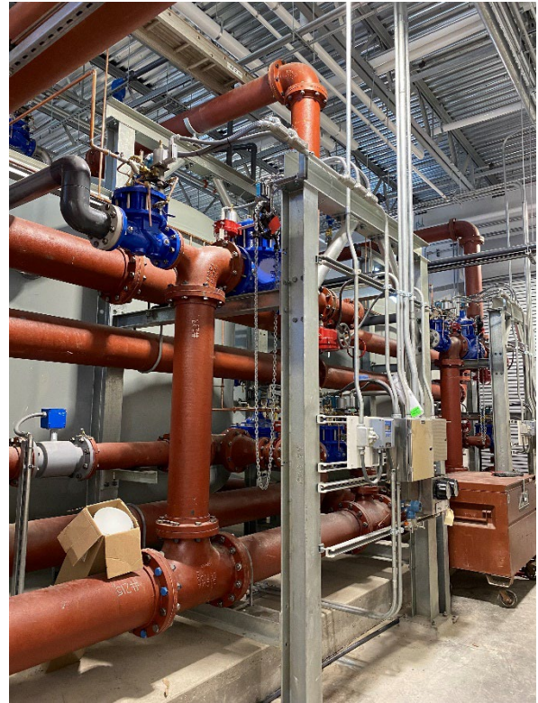
Figure 3: Work continues on the Pudding Hill Treatment Plant.
