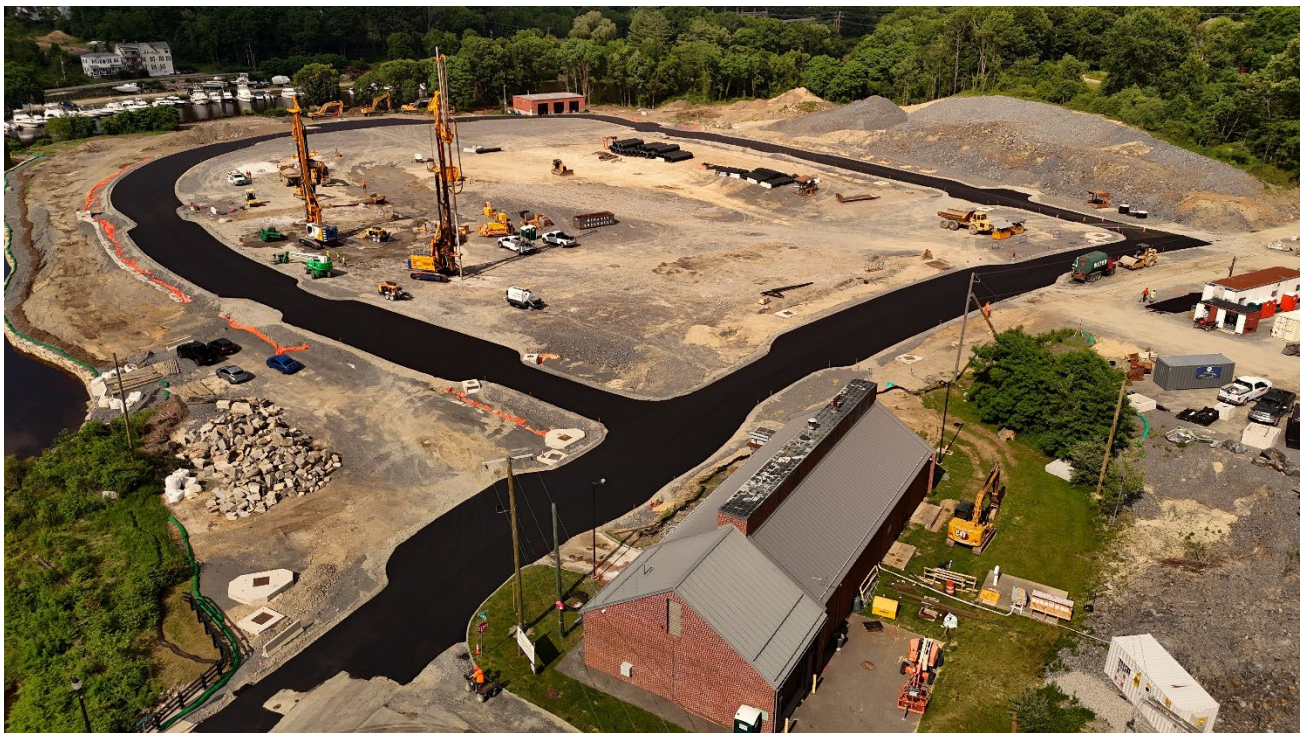
Figure 4: Base course pavement has been installed at the waterfront redevelopment site.
