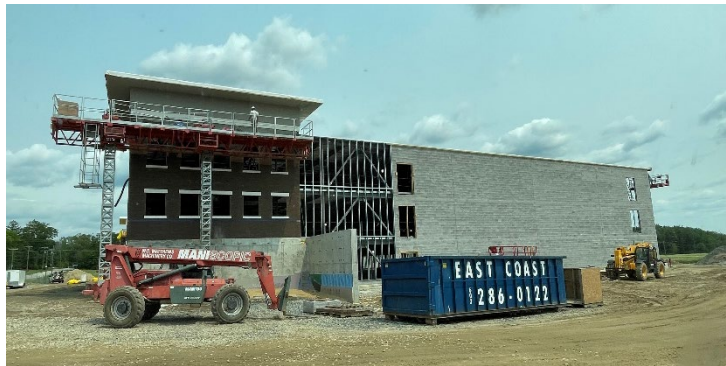
Figure 8: Brick installation on the future Bluebird Storage on Littleworth Road.
