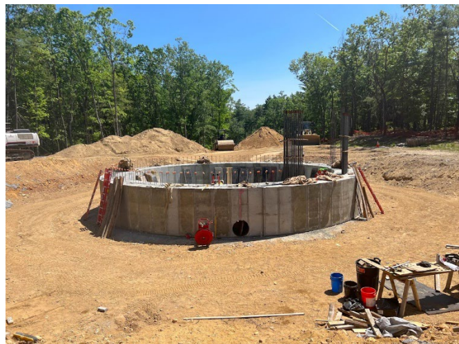
Figure 4: Foundation Ring Wall for Smith Well Road Elevated Tank
