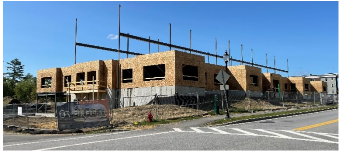
Figure 8: Sitework at residential project at 757 Central Ave.
