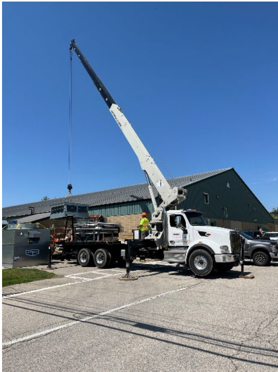
Figure 15: Ice arena cooling tower replacement.
