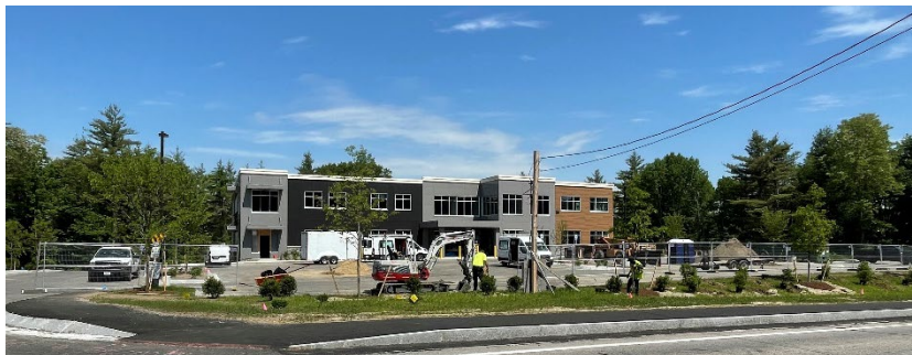
Figure 19: New medical office building on Durham Rd is nearing completion.
