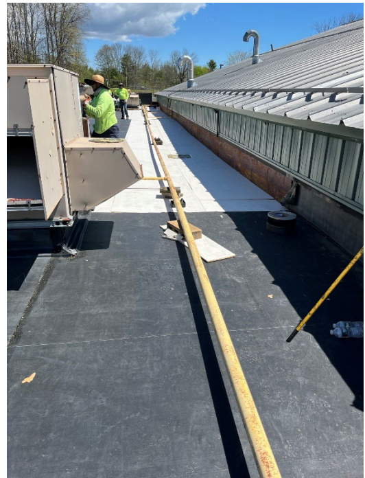
Figure 16: Ice arena roof replacement.
