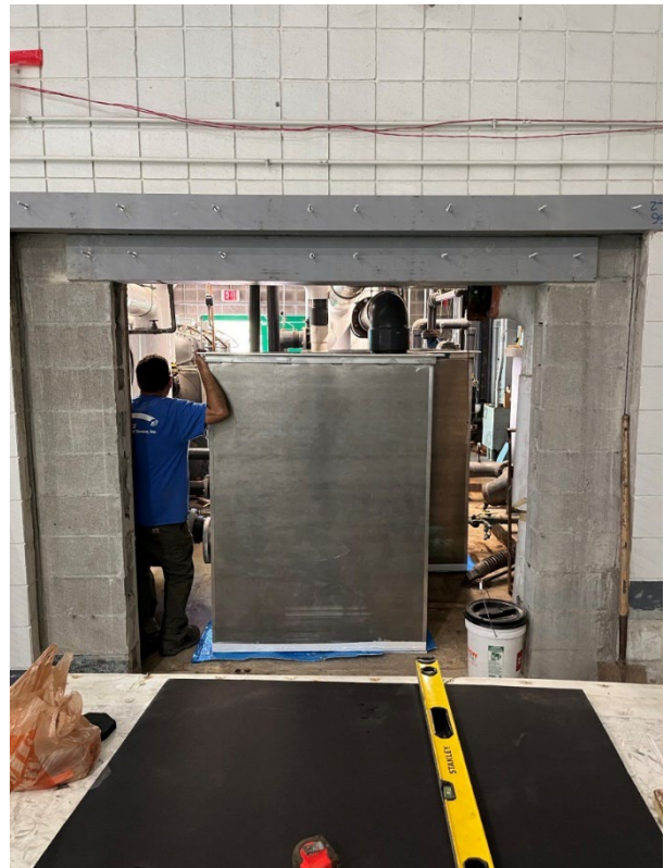
Figure 14: Glycol tank removal in progress.
