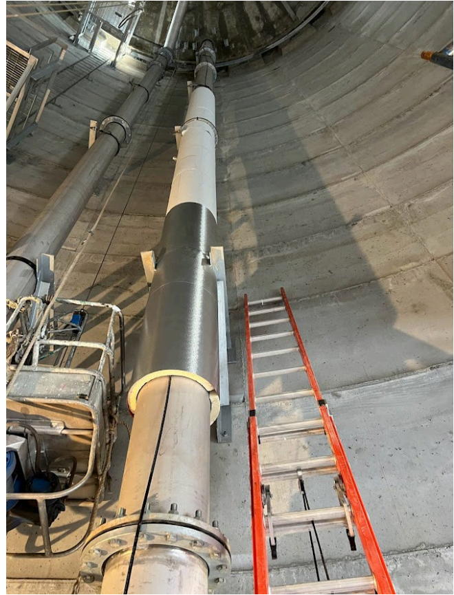
Figure 9: Interior fit up of the new elevated storage tank near Exit 9.
