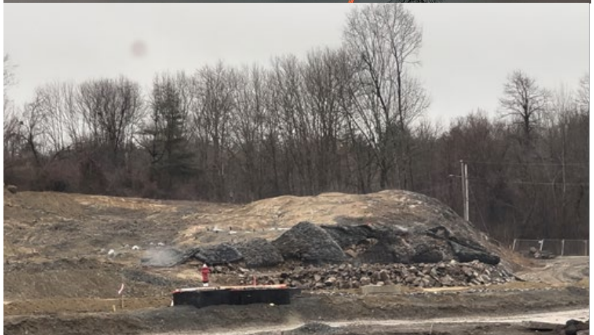
Figure 8: Sitework and blasting continues on the waterfront.
