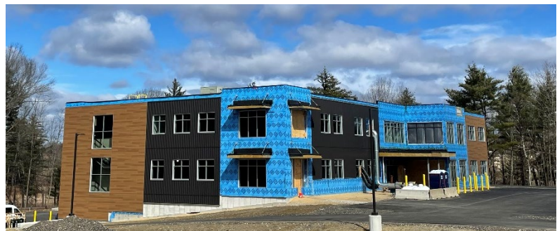
Figure 14: Medical Office Building on Durham Rd.
