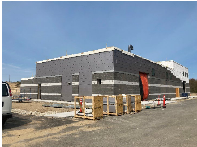
Figure 4: Putty Hill Treatment Plant
