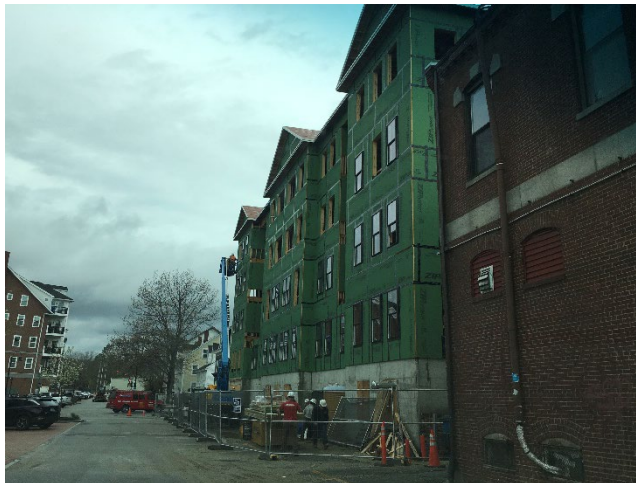
Figure 11: Progress at Courthouse Redevelopment on First St.
