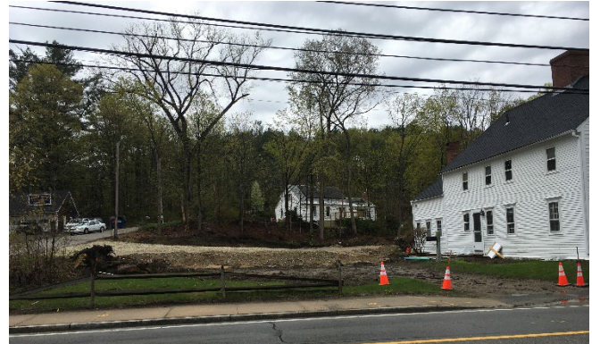
Figure 10: Sitework at residential project at 757 Central Ave.
