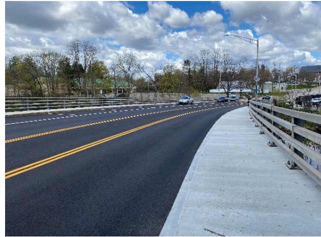
Figure 2: Chestnut Street opened to vehicles and pedestrians 3 weeks ahead of schedule.
