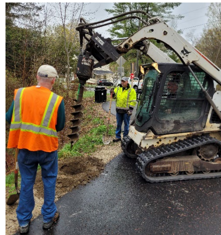
Figure 8: City crews install the Community Trail Scaled Solar System.
