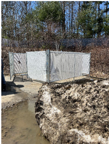
Figure 8: New Willand Pond Warming Center dumpster enclosure.
