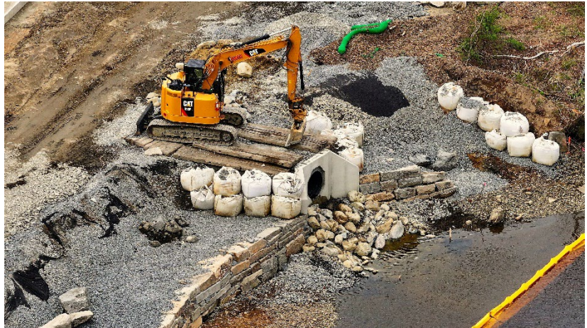
Figure 5: Shoreline granite wall and outfall construction.
