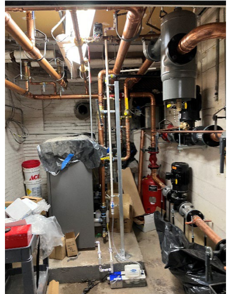
Figure 7: Library Boiler at approx. 75% complete.
