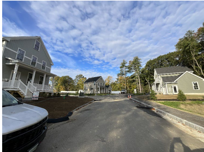
Figure 8: Sophie Dr. nearing completion.
