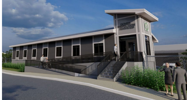
Figure 7: Computer rendering of the new Inspection Services Building at the City's Mast Rd Facility.
