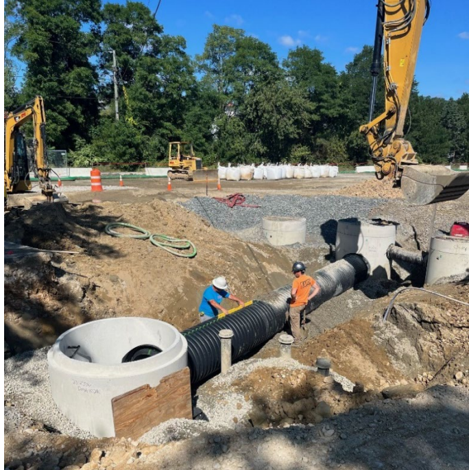
Figure 4: Drainage pipe installation within future waterfront street network.
