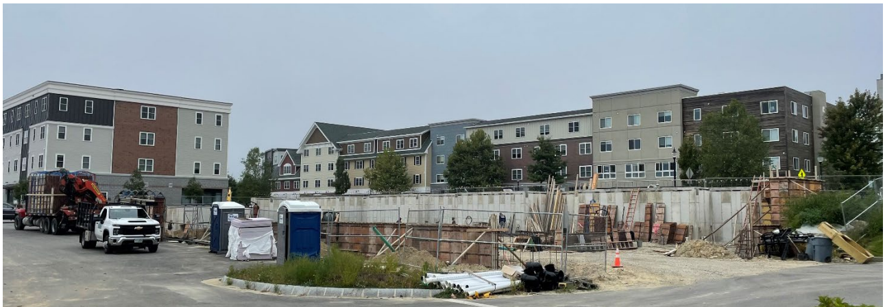
Figure 16: Foundation of 55 Pointe Place is moving along.
