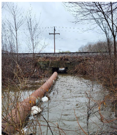
Figure 6: Downstream of the CSX culvert looking back towards Crosby Road.
