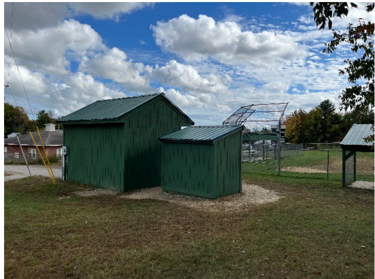
Figure 13: Horne Street baseball field dugouts and facilities received new metal roofs and fresh paint.
