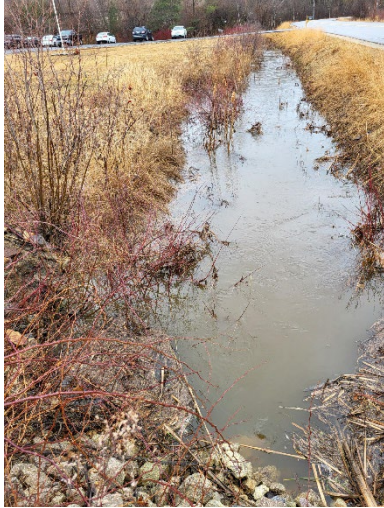
Figure 4: Full drainage channel at Crosby Road.
