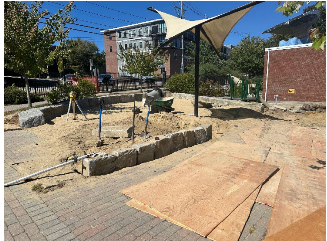
Figure 4: Work on Adventure Park in progress.
