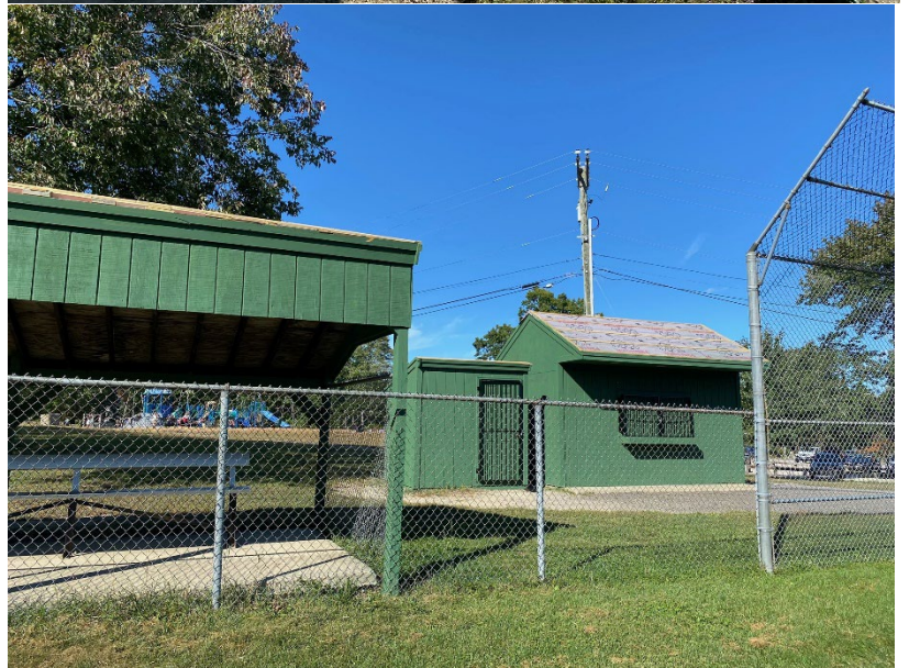
Figure 8: Horne Street School dugout and facility repairs are underway.
