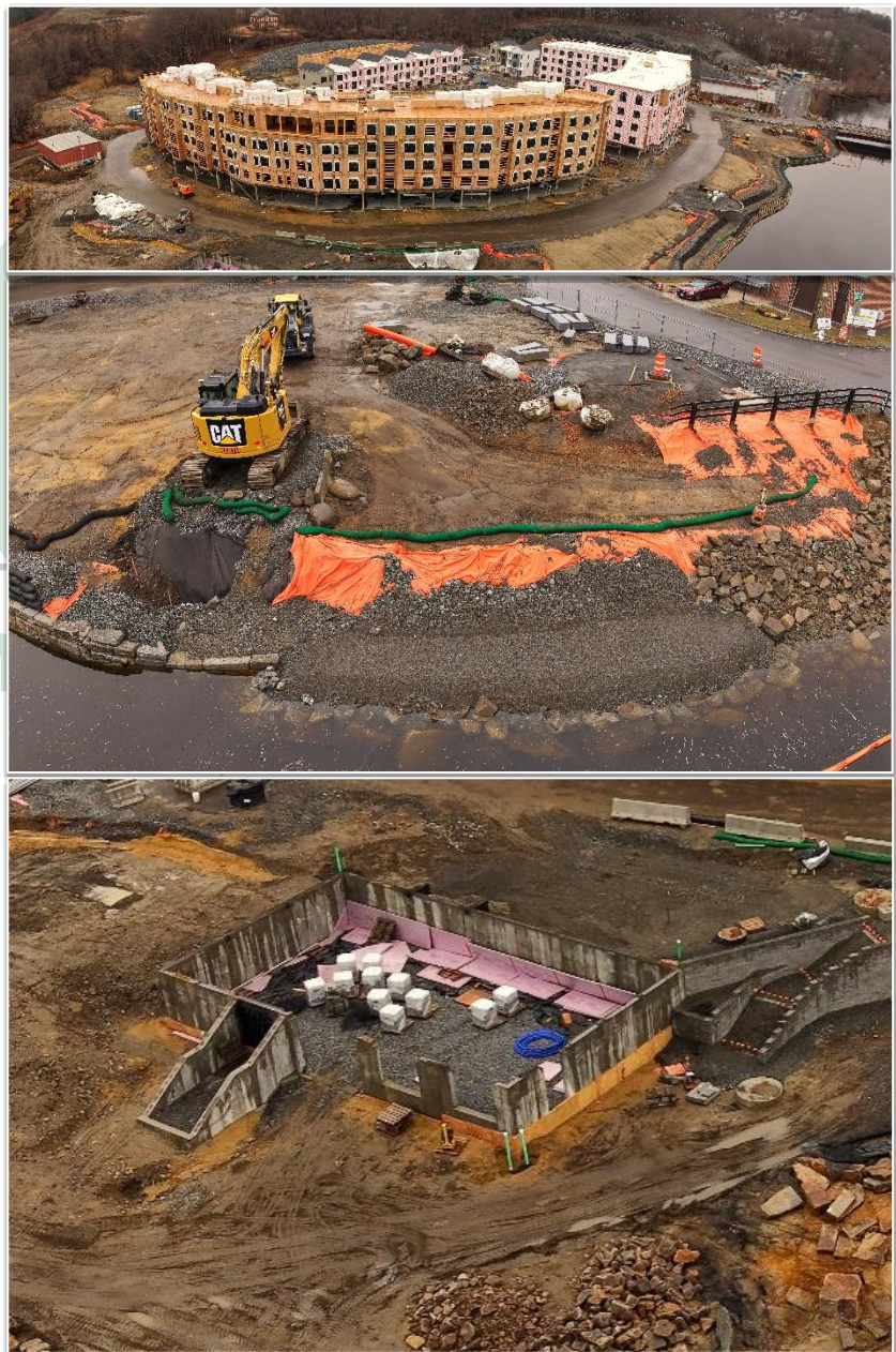
Figure 2: Construction continues on the waterfront as the pavilion takes shape.
