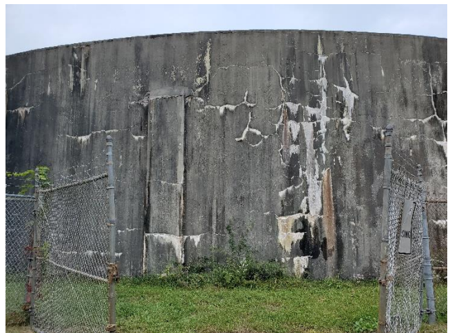
Figure 4: Existing Garrison Hill Tank has been drained and inspected.
