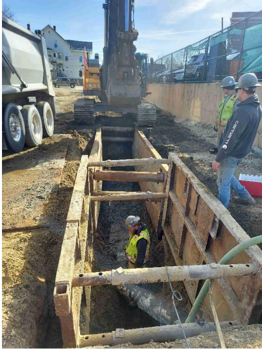
Figure 3: Utility replacement work continues on Angle St.
