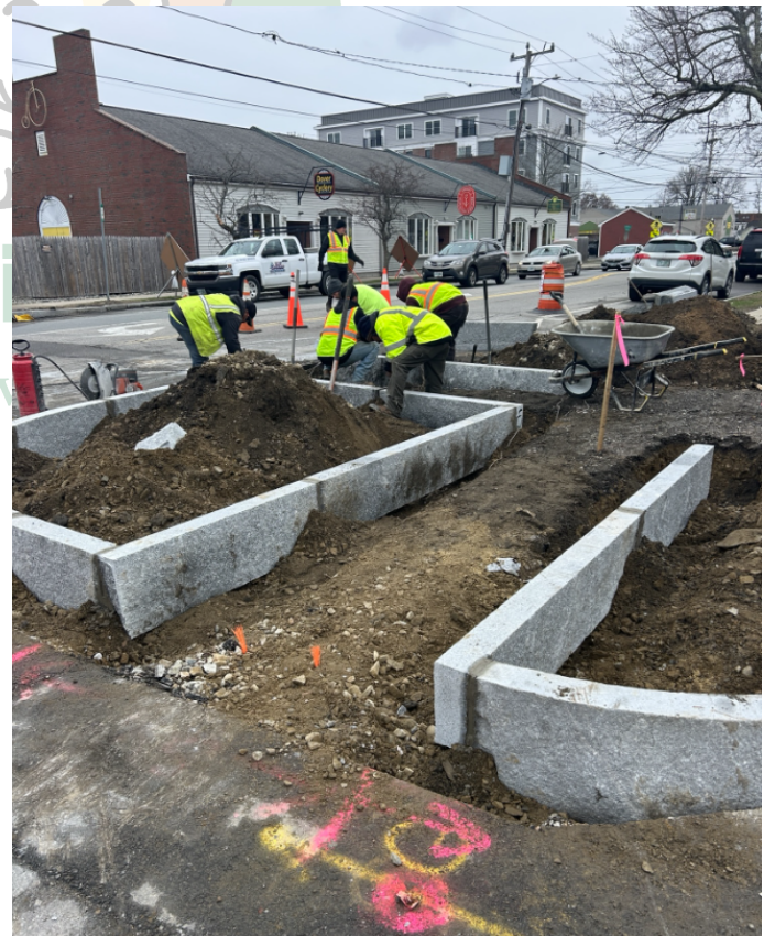
Figure 5: Curbing work at Chestnut and Fifth.
