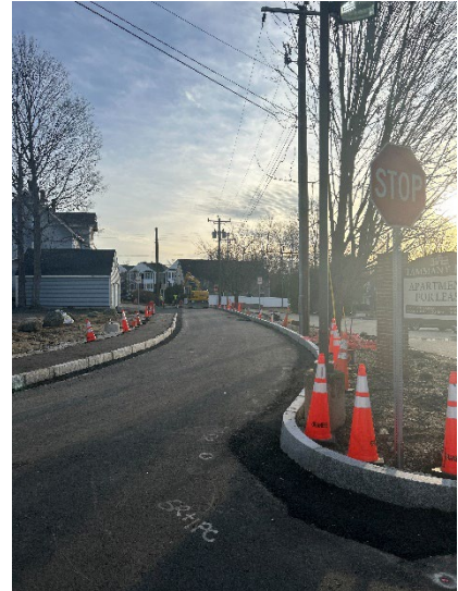
Figure 10: Street improvements on Fifth Street near Tammany Park entrance.
