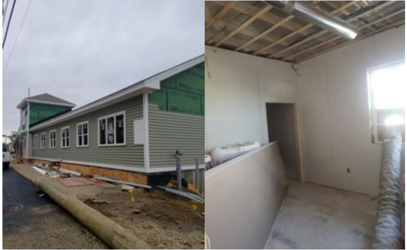
Figure 21: Inspection Services Building on Mast Rd Progress.
