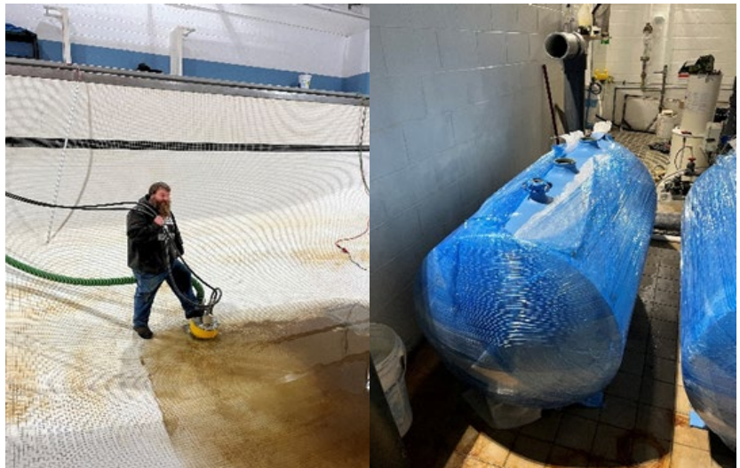
Figure 22: Indoor pool filter replacement work.
