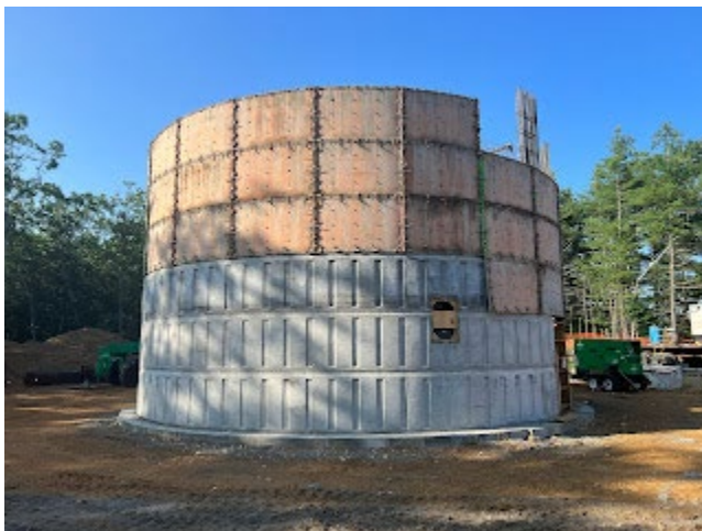
Figure 3: Pedestal for Smith Well Road Elevated Tank
