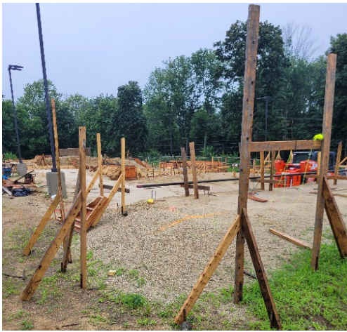
Figure 5: New Dover Skate Park Framing.
