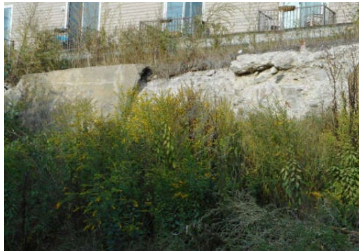
Figure 1: Portland Ave Retaining Wall.
