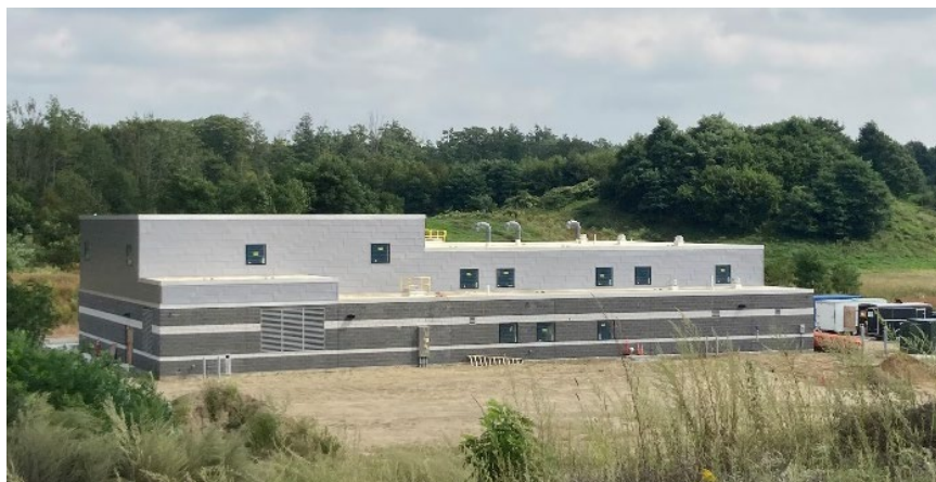
Figure 3: Exterior of the new Pudding Hill Water Treatment Plant.
