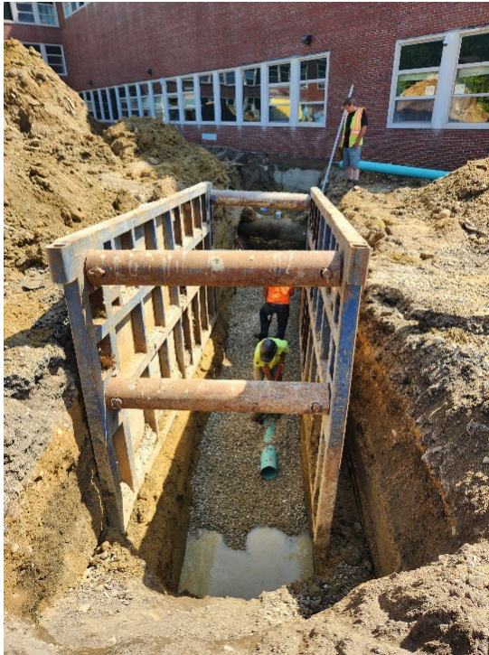
Figure 5: Sewer service reconstruction at Woodman Park School.
