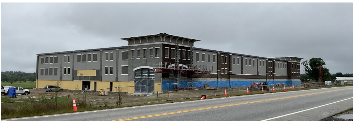
Figure 9: Bluebird Storage on Littleworth Rd.
