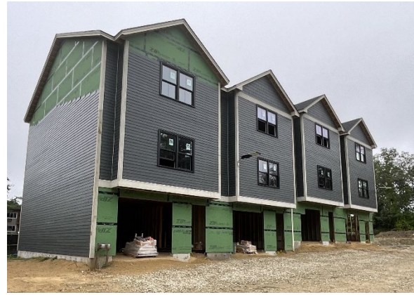
Figure 10: Residential units at 73 Rutland St.
