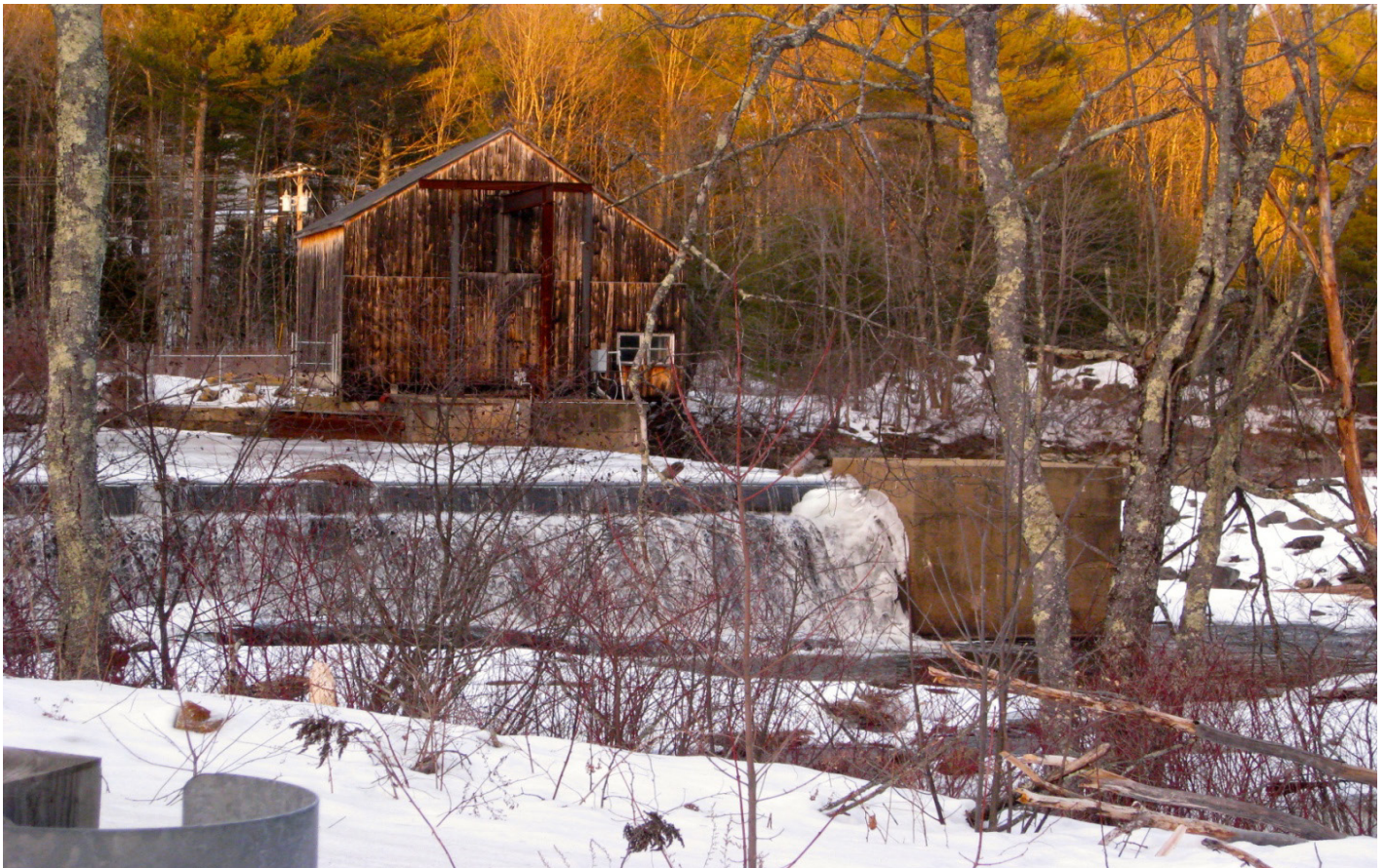
Figure 9. Watson Waldron Dam on the Cochecho River
