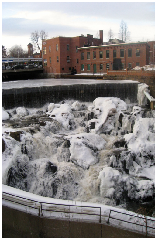
Figure 14. Central Avenue Dam on the Cochecho River
