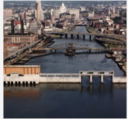
c) Hurricane Barrier
