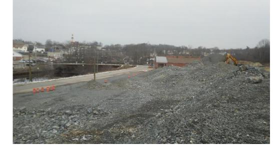
Much of the excavated material will be used be used to raise the elevation of the waterfront site in preparation for future building development. The remaining materials consisting of processed rock and stone dust will be used by the City to construct streets and utilities on the waterfront site as part of the site development process.
