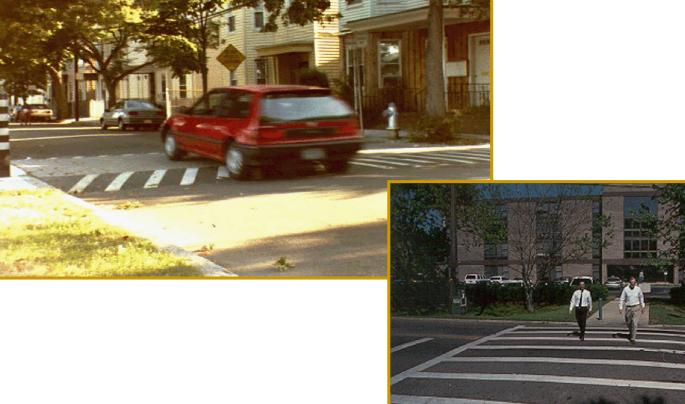
Raised crosswalks are elongated speed humps with a flat section in the
