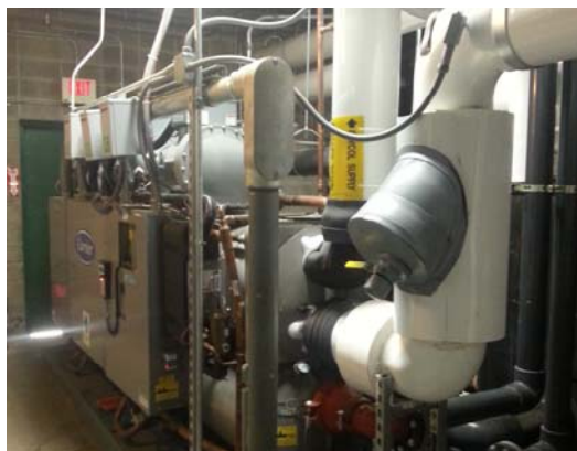
New Electric Chiller Installed at the Ice Arena
