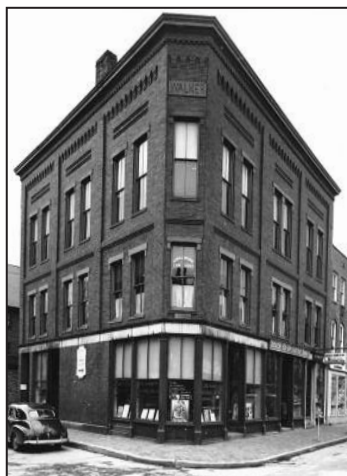
Our Walker Block offices.
