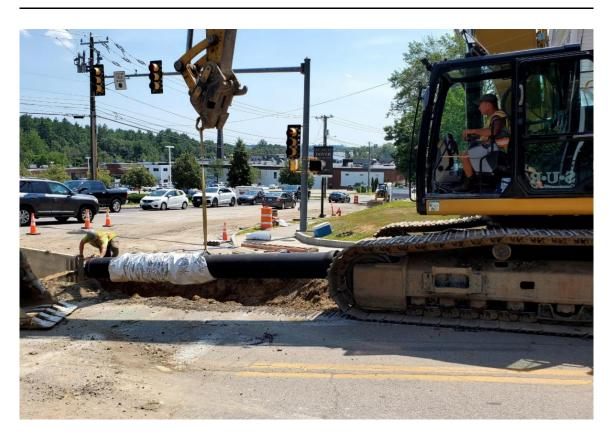
A city contractor is installing a new water main on Oak Street as part of a project to install a new main on Broadway and Oak streets.
